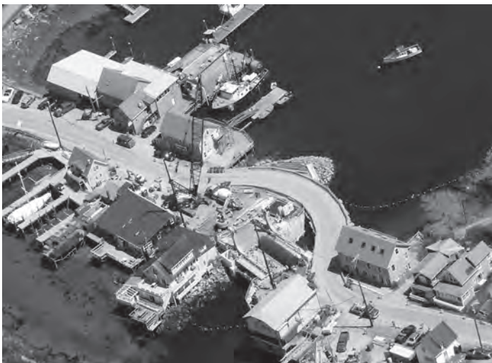
Aerial view with temporary bridge
