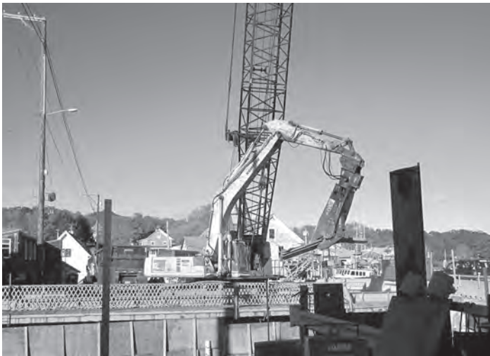
Demolition of the swing bridge begins, 11/2/13/15
