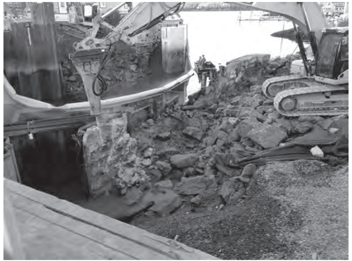
Grinding out ledge, 1/20/15
