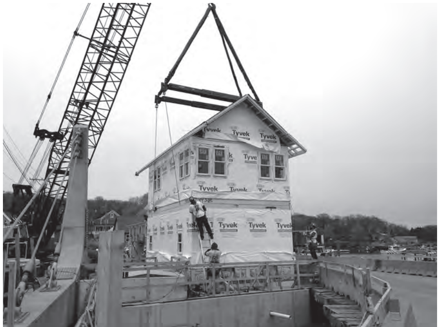
Second story of control house is lowered into place, 5/20/16
