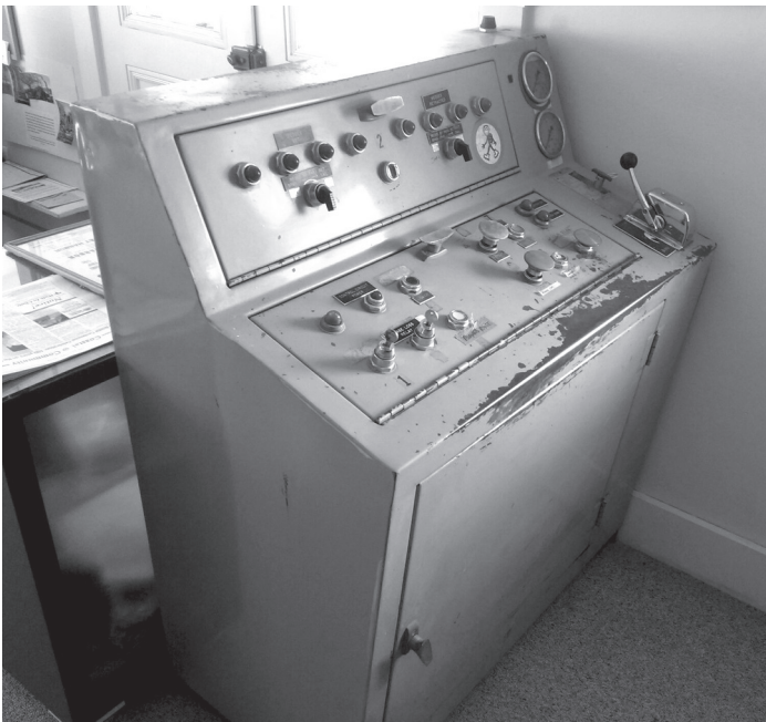
The bridge tender controlled the opening and closing of the 1930 bridge using this console.
